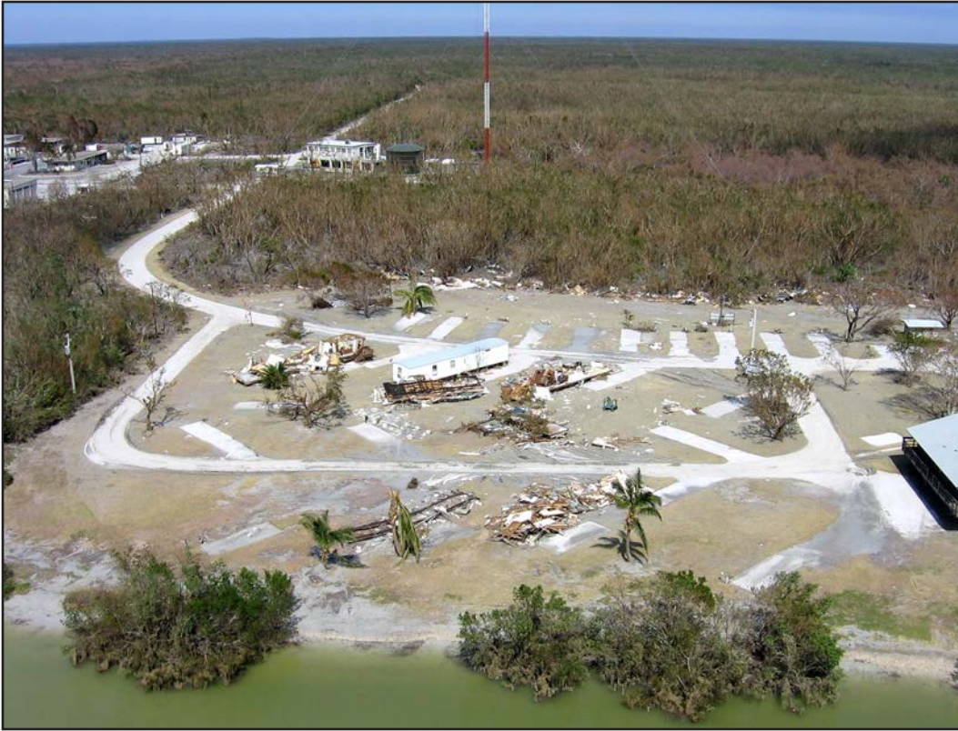
Figure 16-4. Flamingo housing area following Hurricane Wilma, 2005
